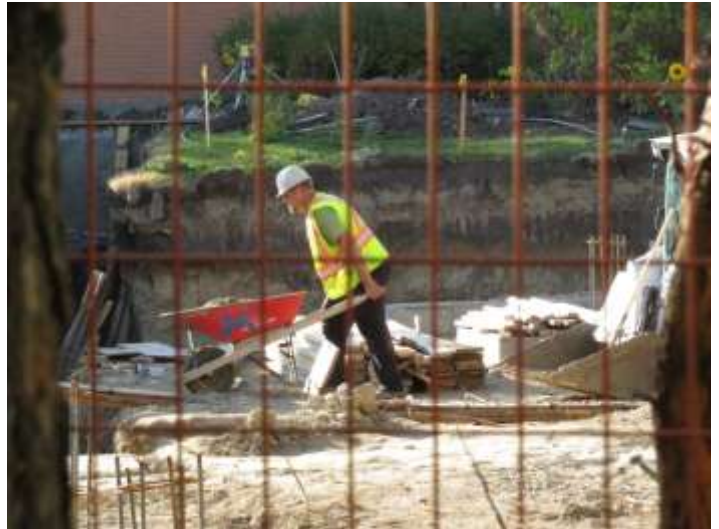
Dumping gravel onto the lower basement floor
