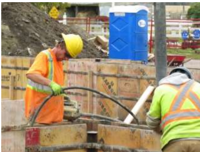
Filling the basement walls with concrete
