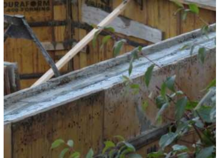
Lower basement floor ready for concrete. Upper basement walls are filled.
