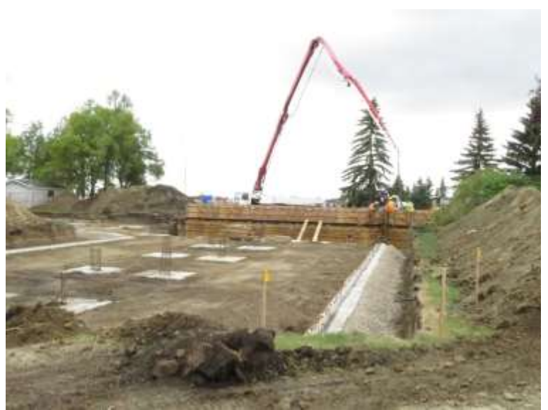
Filling the basement walls with concrete
