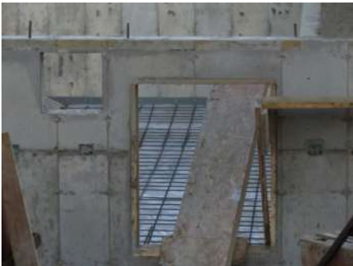
Lower basement floor ready for concrete. Upper basement walls are filled.
