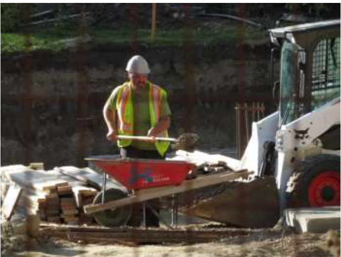
Dumping gravel onto the lower basement floor
