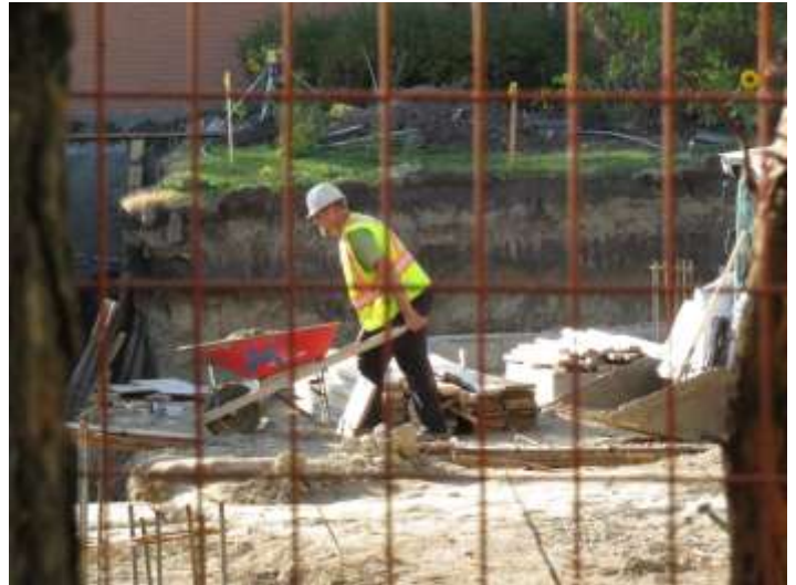
Dumping gravel onto the lower basement floor
