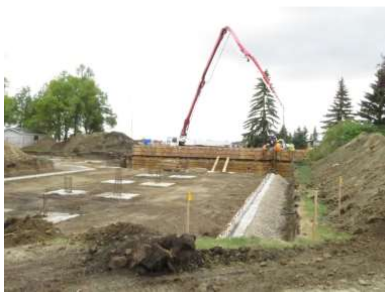
Filling the basement walls with concrete
