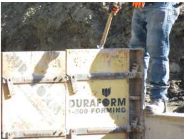
Removing forms from one section of basement and setting new ones for the smaller basement
