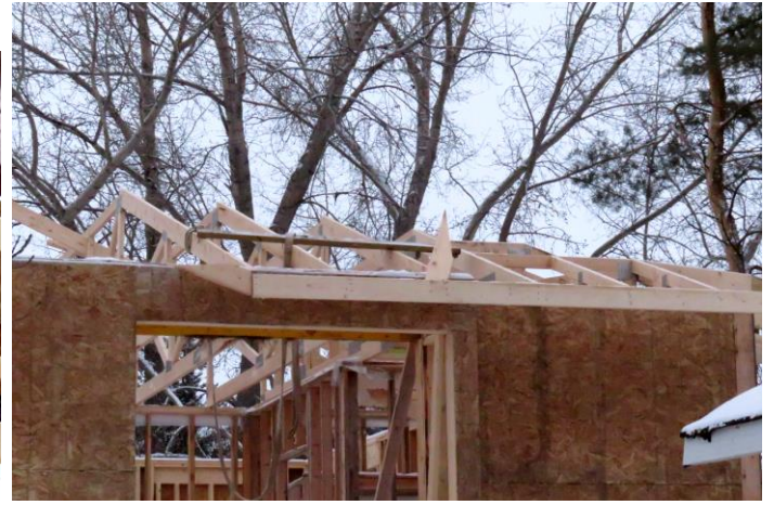
Some of the trusses are up already.
