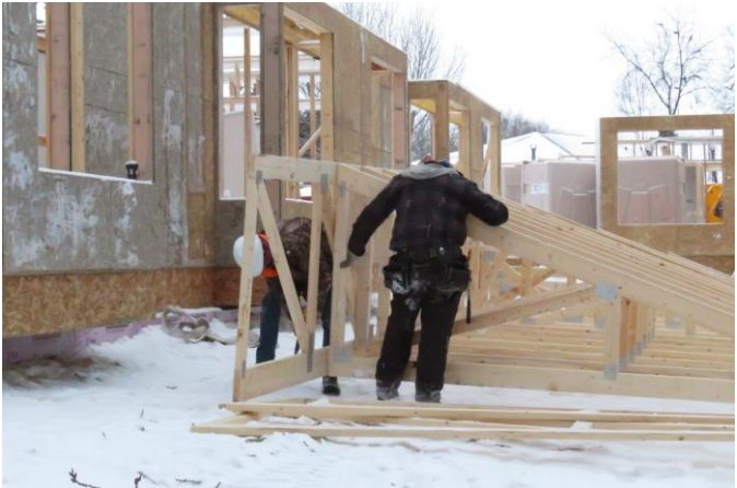
The walls are up on the East Wing. The guys are putting the east wing roof trusses together on the ground.
