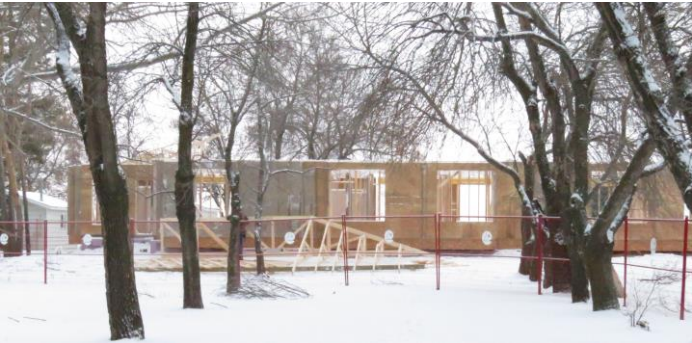
The walls are up on the East Wing. The guys are putting the east wing roof trusses together on the ground.
