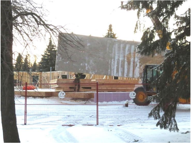
The west wall of the North Wing is up. Lifting and positioning the North wall of the North Wing (on the right). And stabilizing the wall in the photo below.
