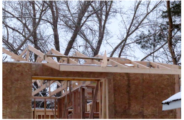
Some of the trusses are up already.
