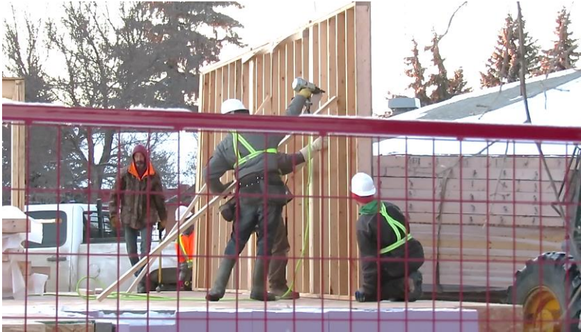
The west wall of the North Wing is up. Lifting and positioning the North wall of the North Wing (on the right). And stabilizing the wall in the photo below.
