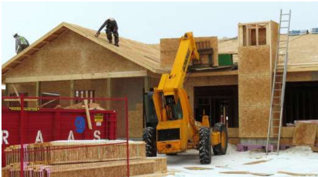
Front entrance taking shape.
