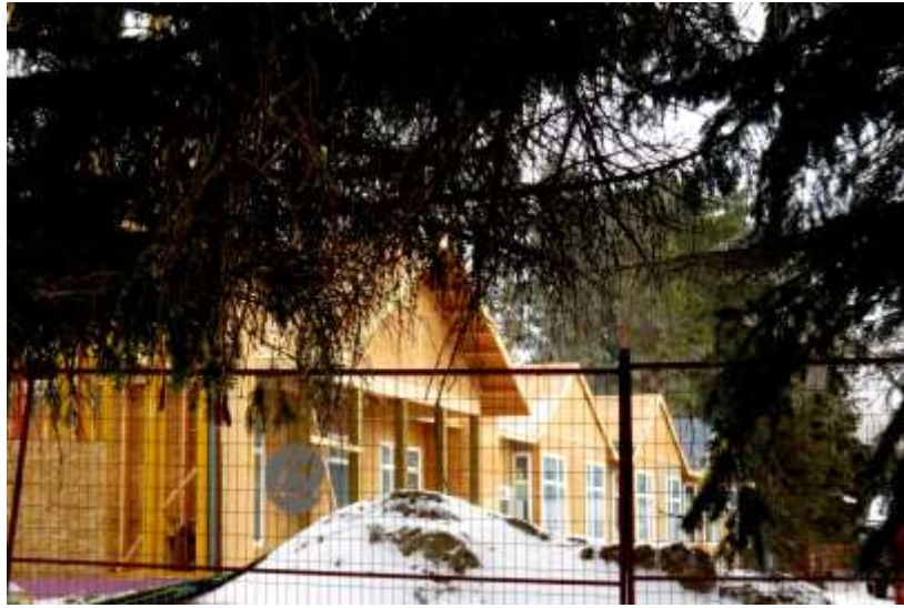
Windows all in on the south side of the building. Looking great!
