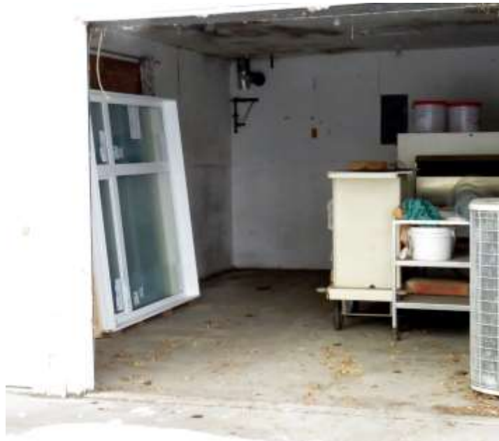
The windows are nearly all gone from the garages!
