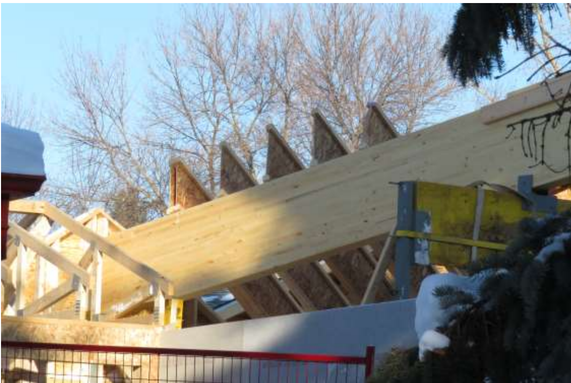
Viewing Chapel roof from the west, looking east.
