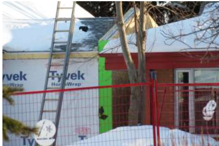
The green indicates the firewall between the Personal Care Home and Pineview
