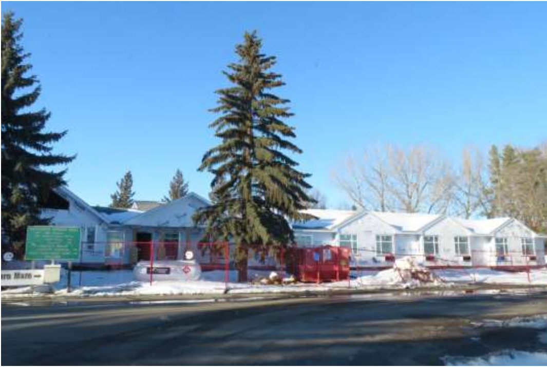
South side looking at the Main Entrance from the stop sign
