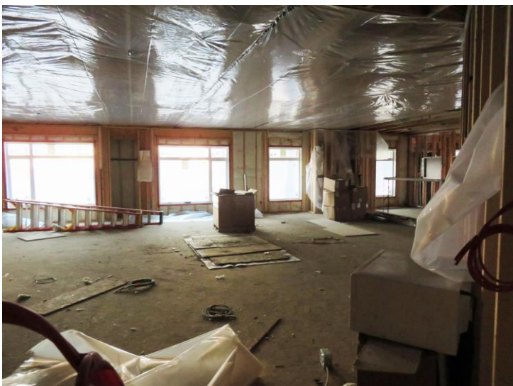
Looking south toward the fireplace area
