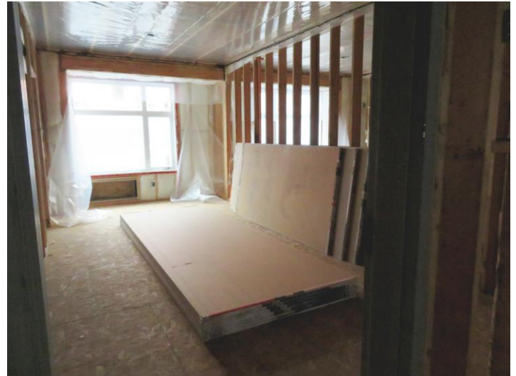
A Room with the drywall waiting!
