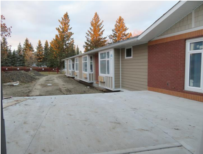
Looking north on the west side of the North Wing
