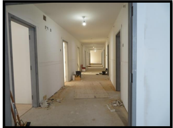
Looking down one of the hallways
