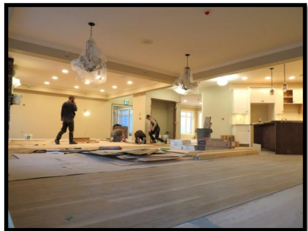
In the “Common and Kitchen Area”—late in the evening installing the flooring
